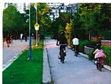
Off street, provide paved paths for bikes only and keep them obstacle-free with clear sightlines.
